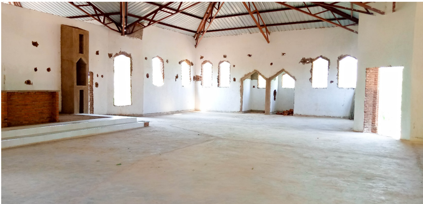
Picture of the left wing of the church showing whitewashed walls and floor.
